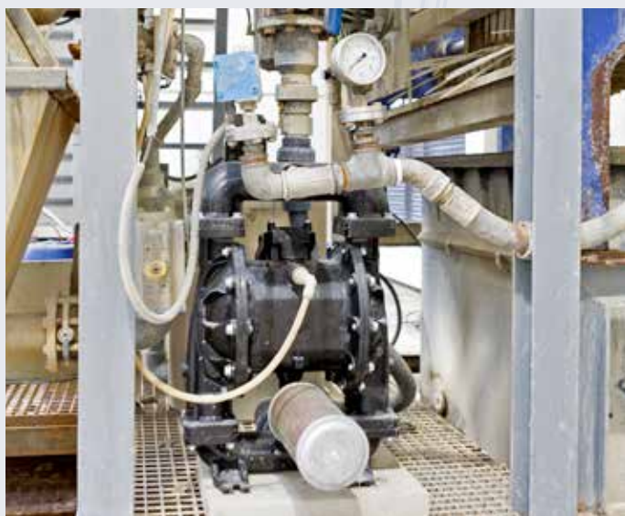
High suction lift reduces pump delivery.
